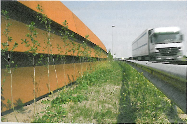
Noise barriers by MTD landscapsarchitecten.
